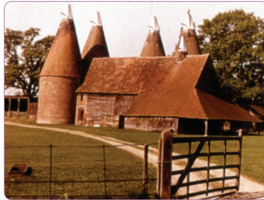
LEFT Schematic drawing showing the workings of an oast. (© National Trust) RIGHT The stowage attached to the kilns may be part of an earlier timber-framed oast. (© Kent County Council)
