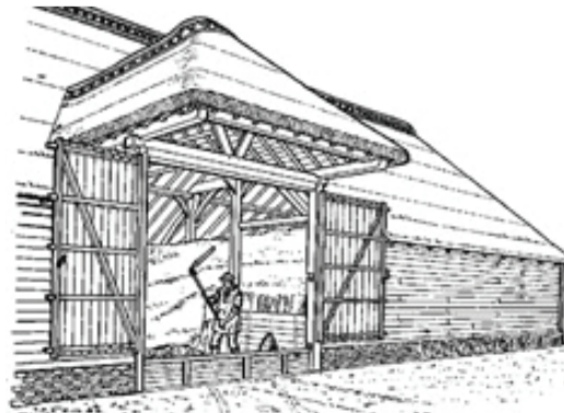
LEFT A late 18th century barn in the Greensand, with its distinctive central door to the threshing bay. The low-pitched and half-hipped roof is typical of this date (Wealden Greensand). (© Bob Edwards)
