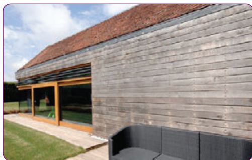
Example of a non-domestic opening in a traditional farm building
