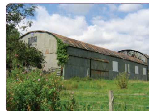
A typical mid 20th century shed, with a curved profile to the roof which resembles those used for iron-framed Dutch barns that date back to the late 19th century. (© English Heritage)
