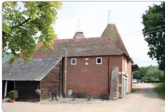
LEFT Large-scale industrial kilns near Goudhurst. Square kilns were built for a time in the 19th century. (© Bob Edwards) RIGHT This brick stowage has an internal timber-frame. (© Bob Edwards)
