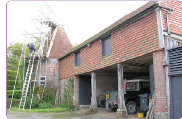
LEFT A cartshed in its typical roadside position. (© English Heritage)
