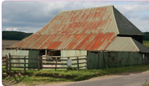
Small 3-bay barns, built on the smaller farms in the High Weald and around the coastal marshes, have rarely survived. These show a barn on the Hoo Peninsula (left) and one on the edge of Romney Marsh. (© Bob Edwards)
