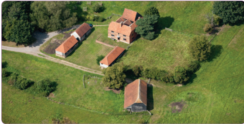
This group in the Low Weald has the house facing into a yard. To the rear of the house is a back kitchen, illustrated on p.33, and in front of the yard is a barn with a lean-to for cattle.(© English Heritage NMR 27205-005)
